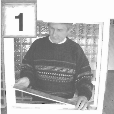
1 Place sill infill in bottom of frame.
