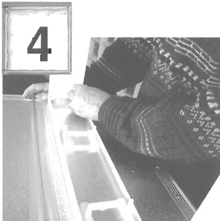
4 Place a cut "T" connector in the bottom corners of the frame on top of the sill infill, with the open end against the expansion material.
