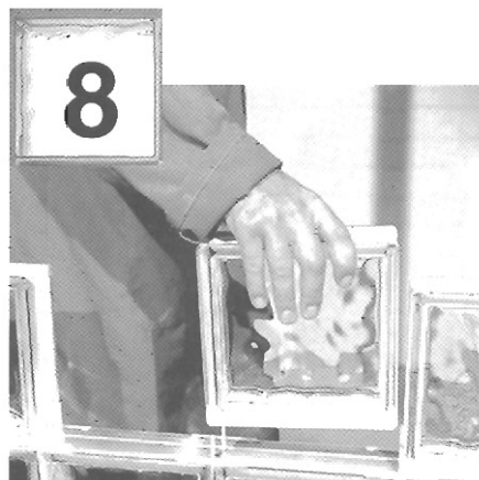
8 Place the next row of glass blocks and then repeat steps 5, 6 and 7 until one stiffener bar and one row of blocks remains to be installed.
