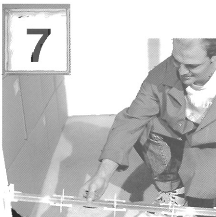
7 Place the stiffener bar, with connectors, onto the first row of glass blocks.
